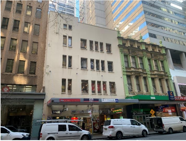
Figure 23 The principal northern Hunter Street façade
