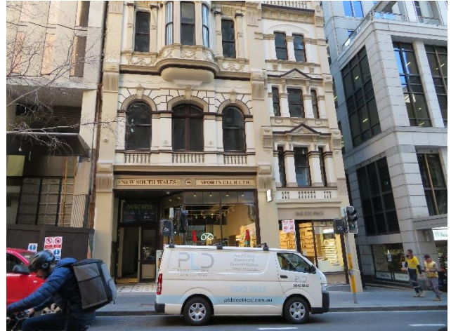
Figure 38 Part view of the former Sports Club (Hunter Street)
